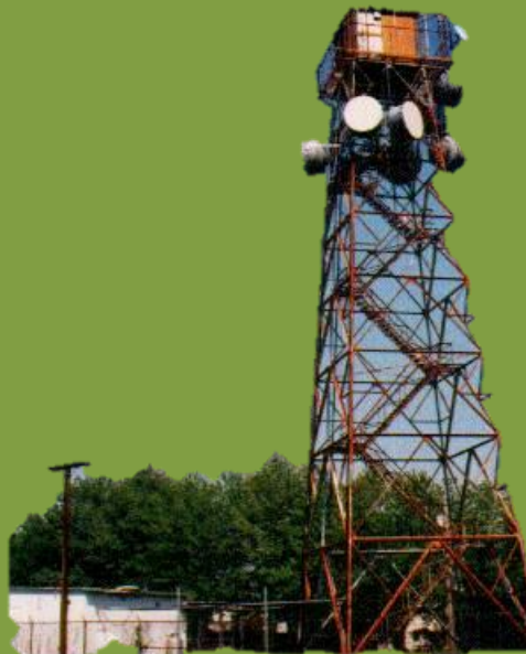
Existing Analog Repeater
